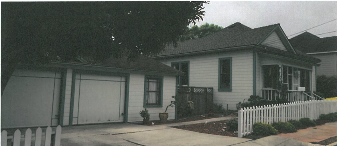
VIEW FROM THE NORTH WEST
