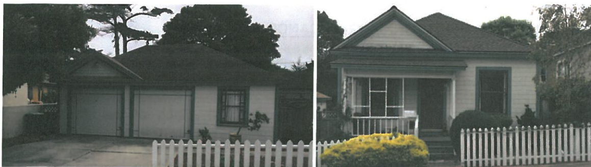
WEST ELEVATION – 213 GRANITE STREET (COMPOSITE PHOTO)
