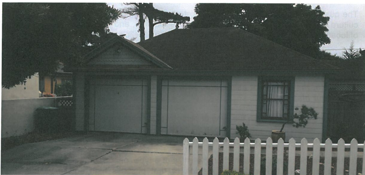
DETACHED GARAGE – NON-HISTORIC
